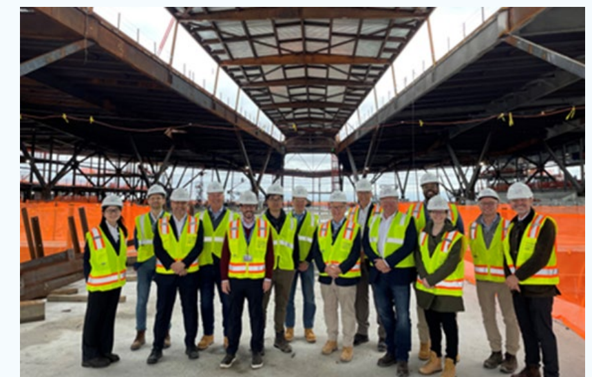
State infrastructure coordinators visit The New Terminal One at JFK
